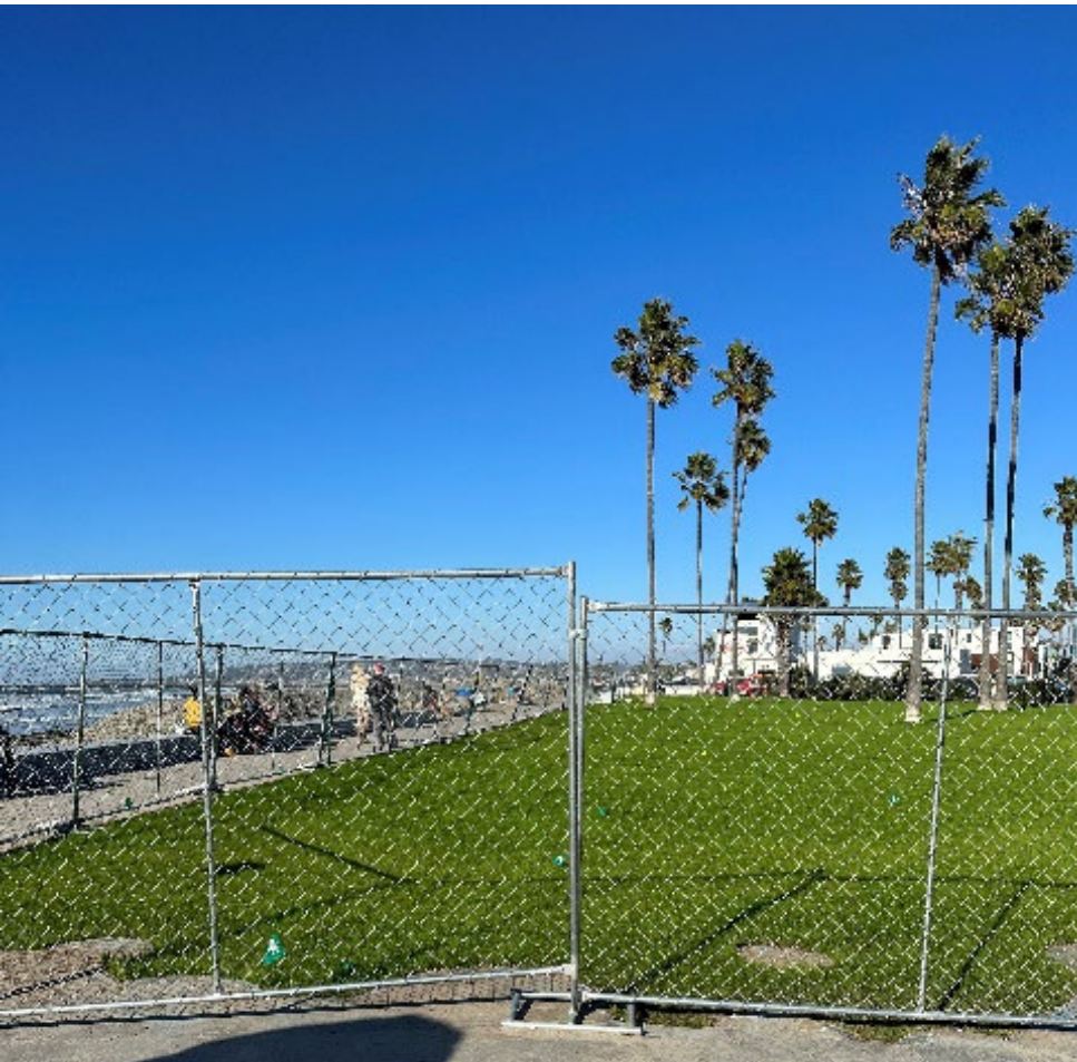
Progress in January 2024
